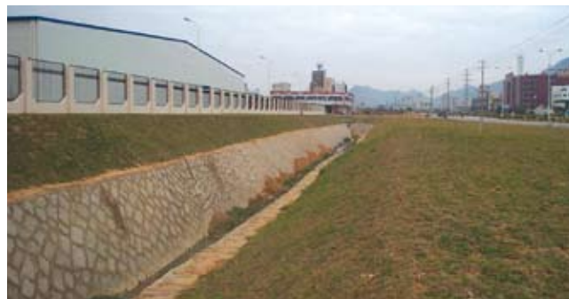
Figure 3: Example of a site platform being elevated higher than the surrounding
