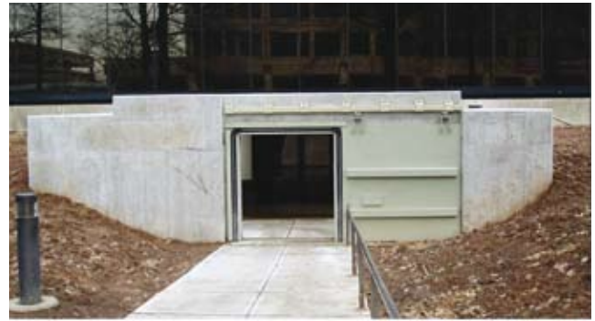
Figure 4: Example of a flood door to a below ground space
