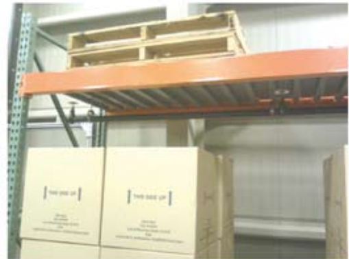
Figure 2: Storage racks with an installed in-rack automatic sprinkler system
